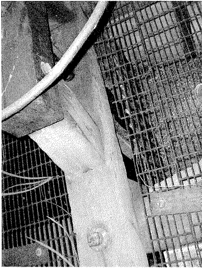
Description: Floor grate and weir at downstream gatehouse.
